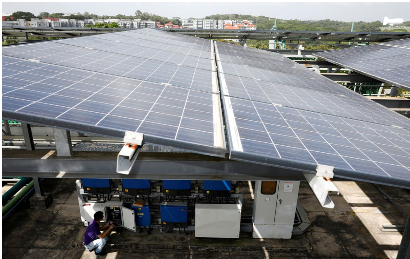
An Electrify SG engineer shows how a PowerPod is installed to record data of photovoltaic solar panels on a rooftop in Singapore, December 18, 2017. Electrify is a Singaporean company that has launched a blockchain-based exchange. Picture taken December 18, 2017. REUTERS/Edgar Su
